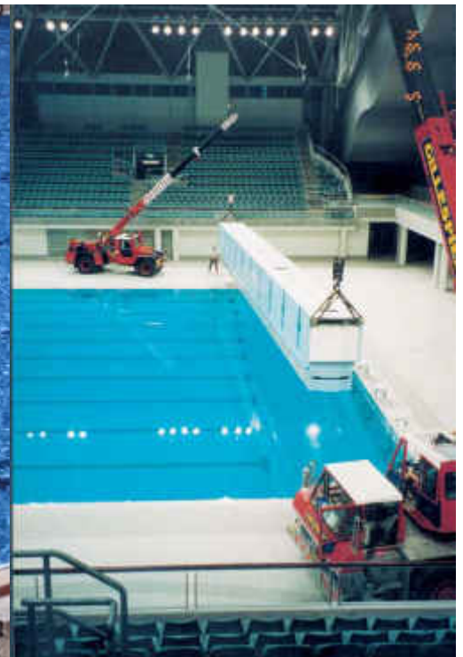
Anti Wave Movable Bulkhead Installed • Instalation
