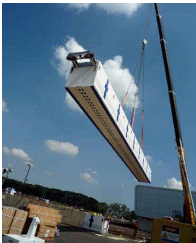
Bulkhead Installation • Melbourne • Australia • 2009
