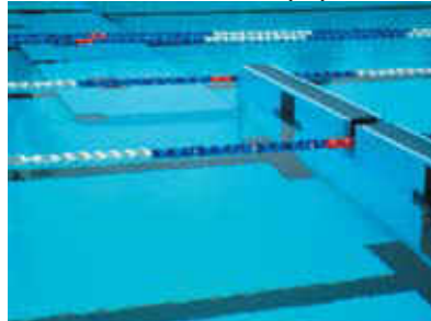
Bulkhead locked in 'up' position
