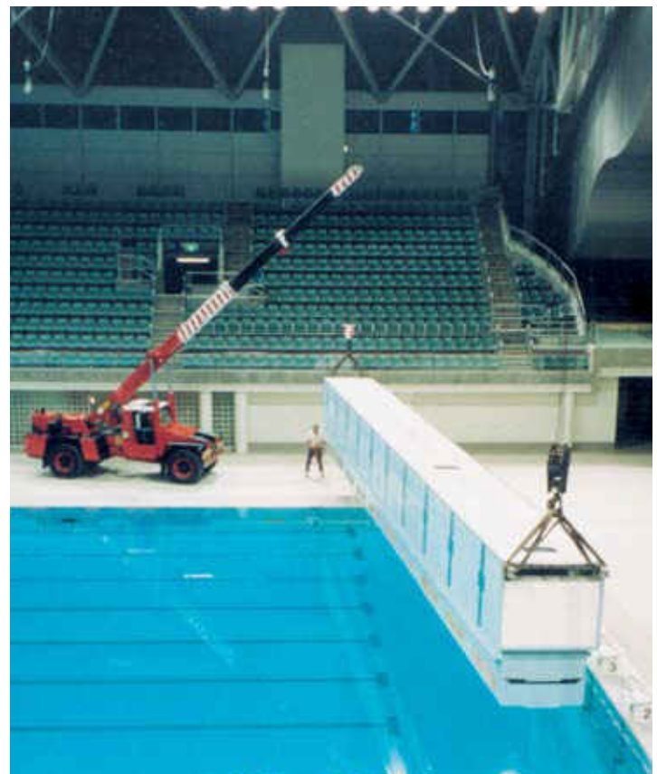
Bulkhead Installation
